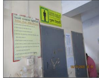
Photo of the sanitary facilities Workers Toilet area.JPG
